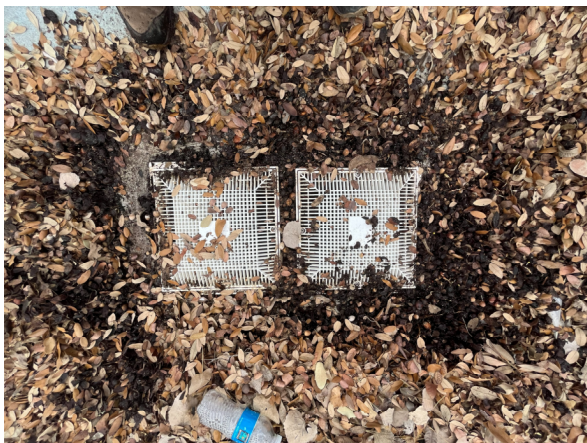
Photo #29 View of the 12" x 12" domed main drains (four (4) instances).
