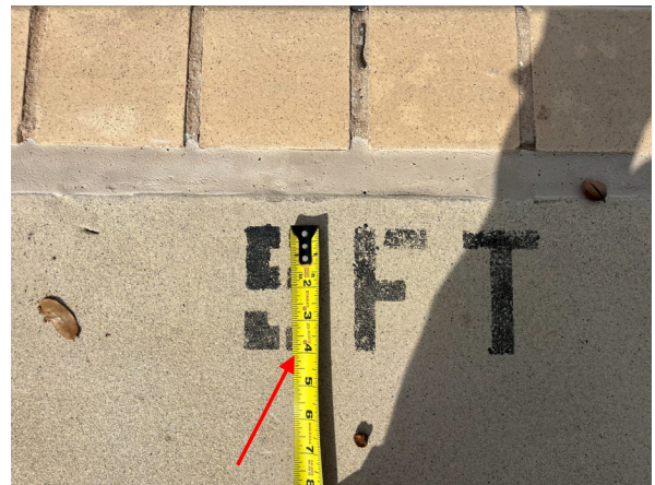
Photo #4 Example view of a 4" tall depth marking on the Lap Pool deck.
