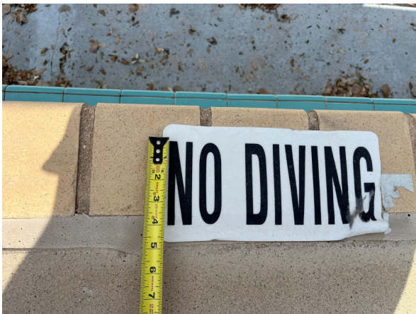
Photo #5 Example view of 4" tall "NO DIVING" sticker at the ramp entry of the Lap Pool.
