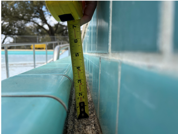
Photo #19 View of the gutter trough that runs around the perimeter of the Lap Pool.
