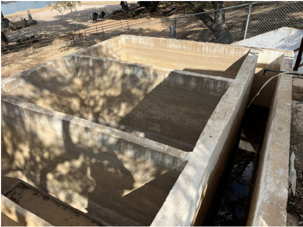
Photo #34 View of existing Lap Pool vacuum sand filter pits.
