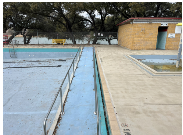
Photo #6 View of the Lap Pool ramp entry.
