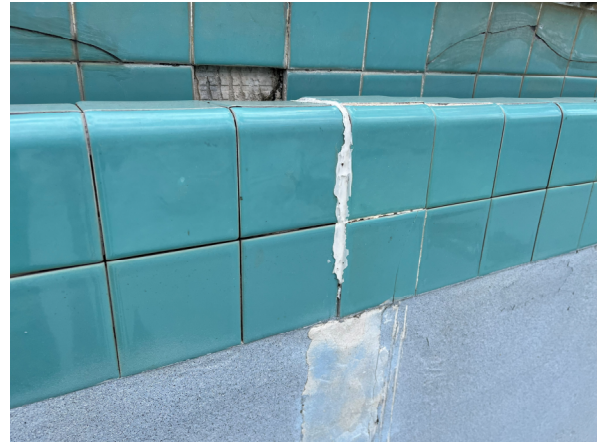
Photo #26 Example view of cracking and chipping of the Lap Pool waterline tile throughout the perimeter.
